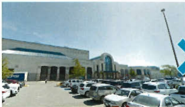
Existing Surface Parking
