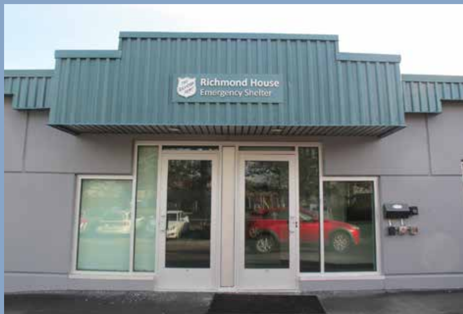
ABOVE: THE NEW EMERGENCY SHELTER PROVIDES SAFE AND SECURE SHELTER SPACES IN A SUPPORTIVE ENVIRONMENT FOR UP TO 36 PEOPLE—MORE THAN TRIPLE THE NUMBER THAT EXISTED PREVIOUSLY.
