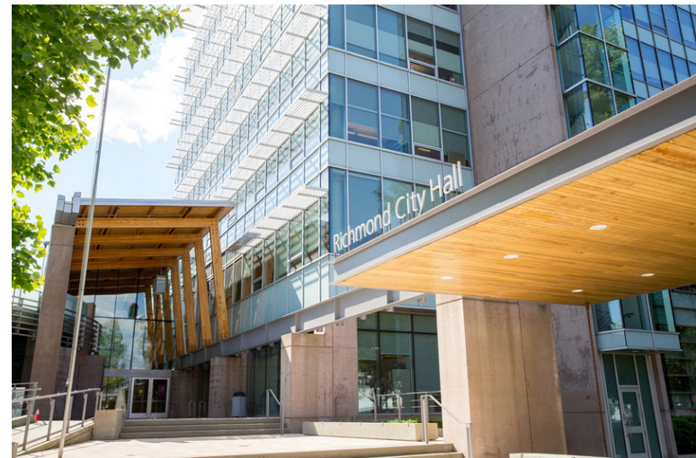
Ensure building envelope detailing sheds the weather in an appropriate manner, and meets energy utilization performance standards.
