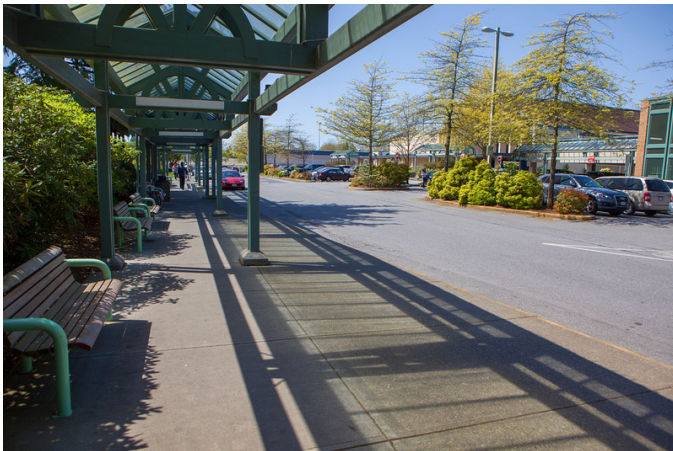
Miscellaneous metals should have a powder coat paint finish.
