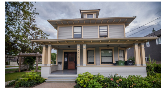
Branscombe House, City of Richmond.
