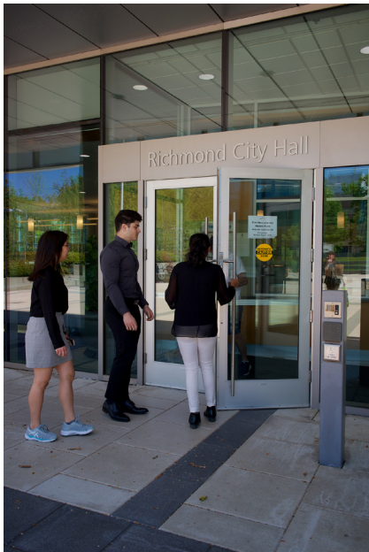
Power - assisted doors to promote accessibility should be installed at building entrances and key interior doors, such as public washroom doors.
