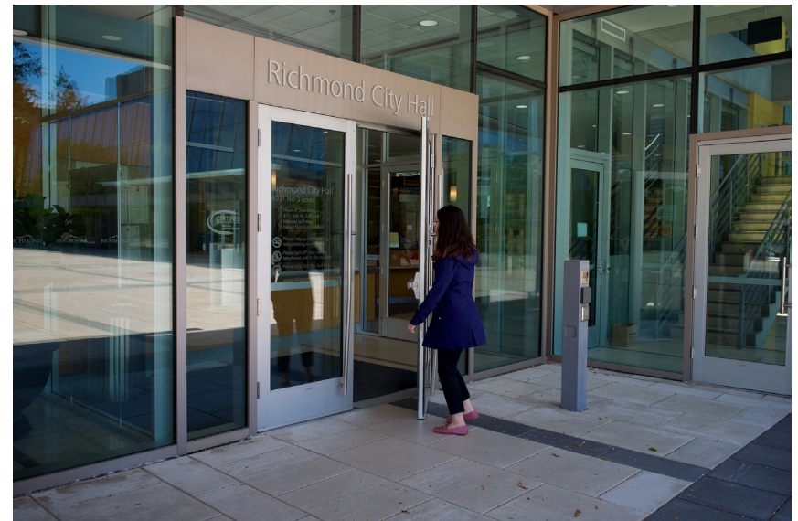
Extensive glazing at doorways into interior lobbies enhances wayfinding and building security. Install security hardware with ease of use and accessibility in mind.
