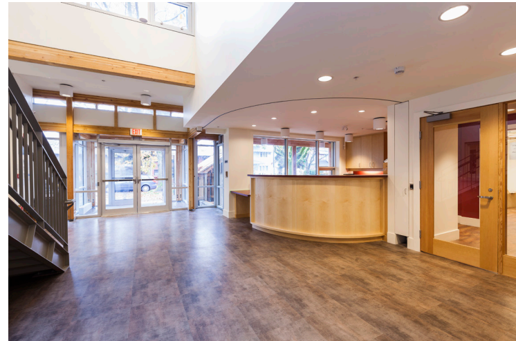
Flooring materials in new builds and renovations should be resilient and highly durable. Vinyl tiles and carpet tiles are preferred to sheet goods, to facilitate replacement and repair. Ensure that 5% extra stock of the total flooring area material is supplied and retained for maintenance purposes.
