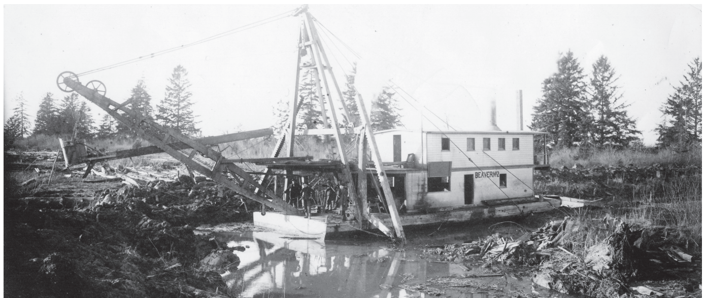
Dyking and the Dredge "Beaver No. 2" in Steveston area, ca. 1905. City of Richmond Archives Photo #1978 14 4
