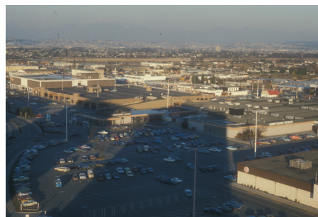
Richmond Square and beyond looking northeast (note shadows of the towers).
