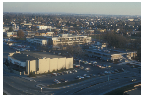
Richmond Square, Municipal Hall and beyond looking southeast.
